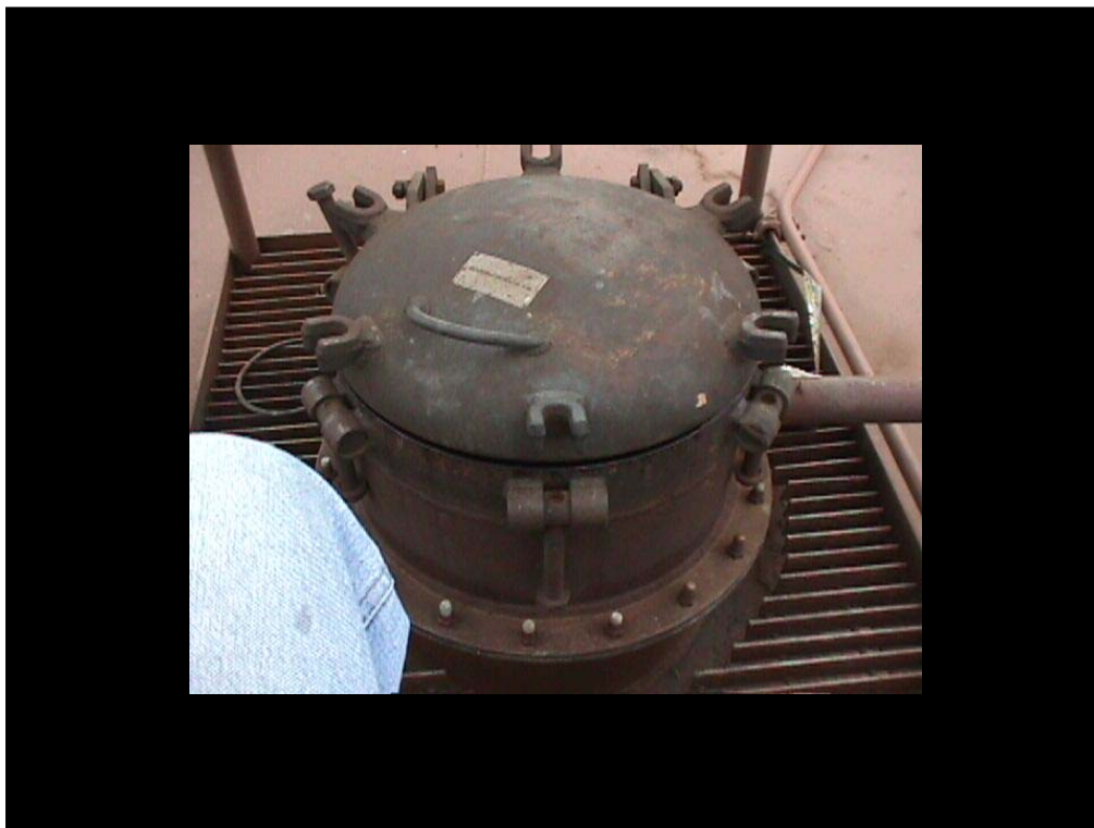
Another unsecured manway. The hatch is not “dogged” down.
